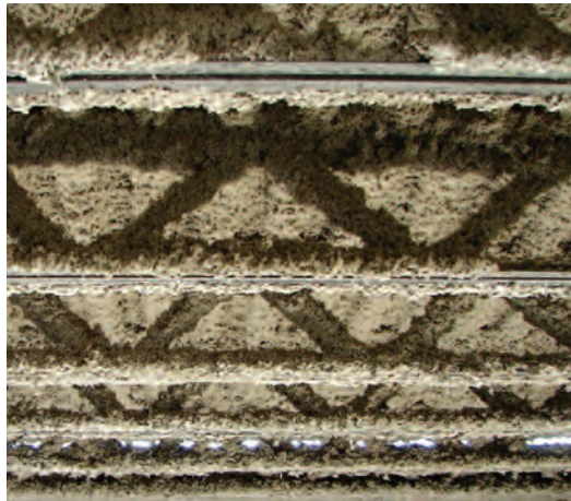
Figure C-4: Fireproofing added to structural steel
